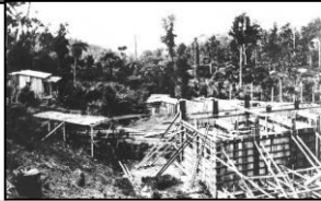
1927 Waitakere Filter Station 1928 Huia Filter Station
